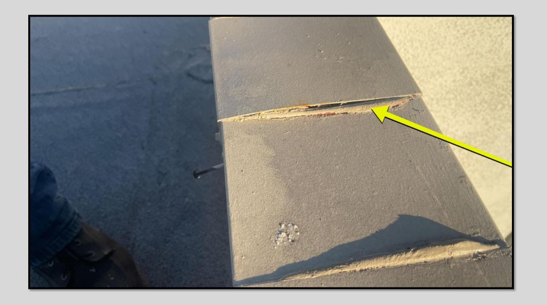
New single-ply PVC membrane addresses exiting roof's weak points
